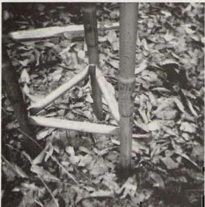
The Dill tower base rests on a large flat rock two feet down and buried in small rocks and well-tamped dirt.
